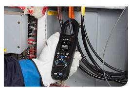
Verify amperage measurements
